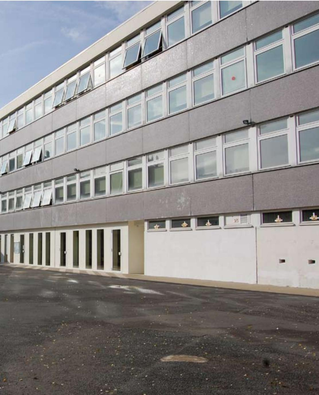
**> MODULES : BÉTON AVEC OU SANS PAREMENT, ET VERRE**
